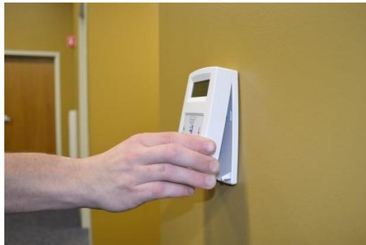
**Step 2:** Push bottom of ExactLogic thermostat in with thumb and forefinger until it clicks back into place
