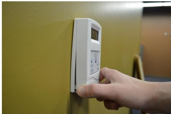
**Step 4:** Once the bottom left corner has popped loose, pull on bottom right corner of ExactLogic thermostat with forefinger until bottom half of thermostat is disconnected from the base of the ExactLogic thermostat.
