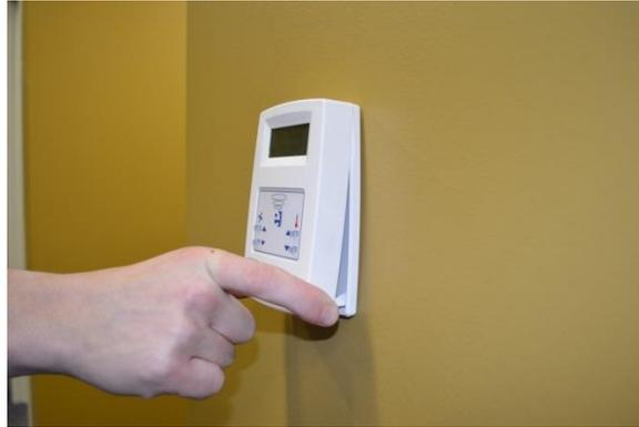
**Step 5:** Pull up on ExactLogic thermostat until the top pops off.
